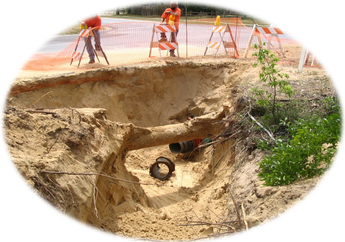
Old Line Removed, Ready for New Line Installation
