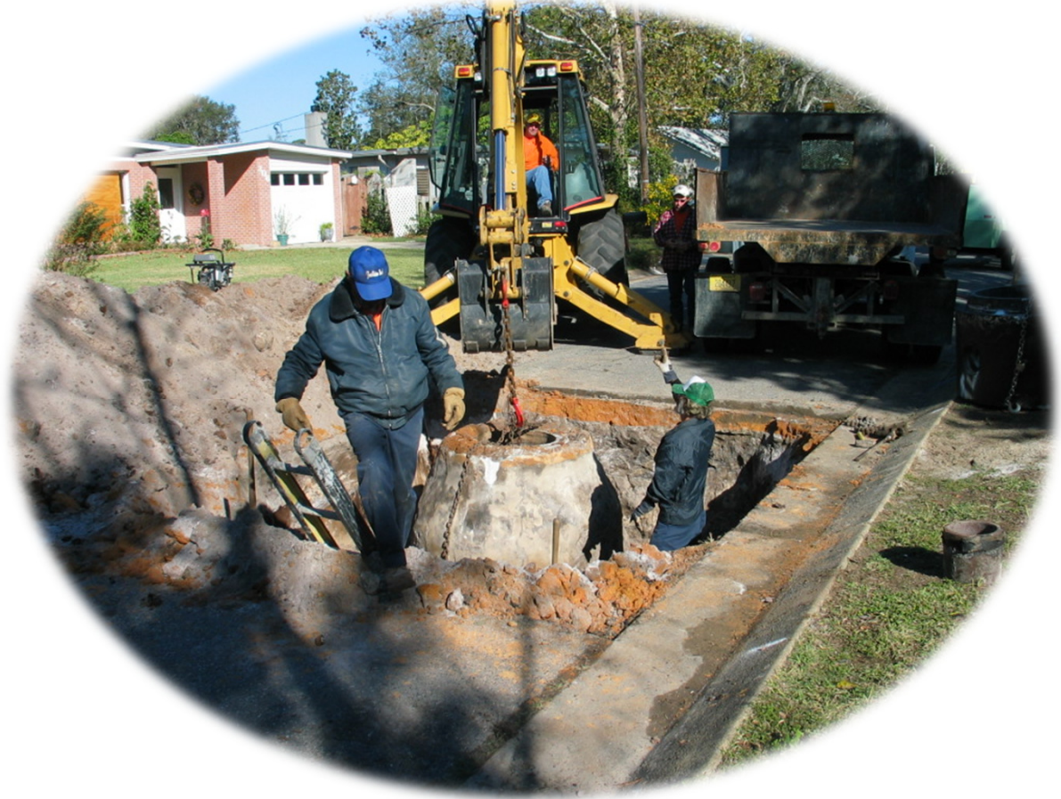
Replacing a Sewer Line
