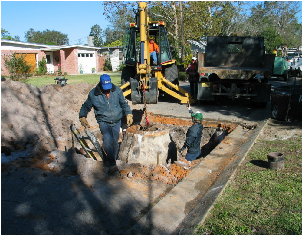
Replacing Sewer Line
