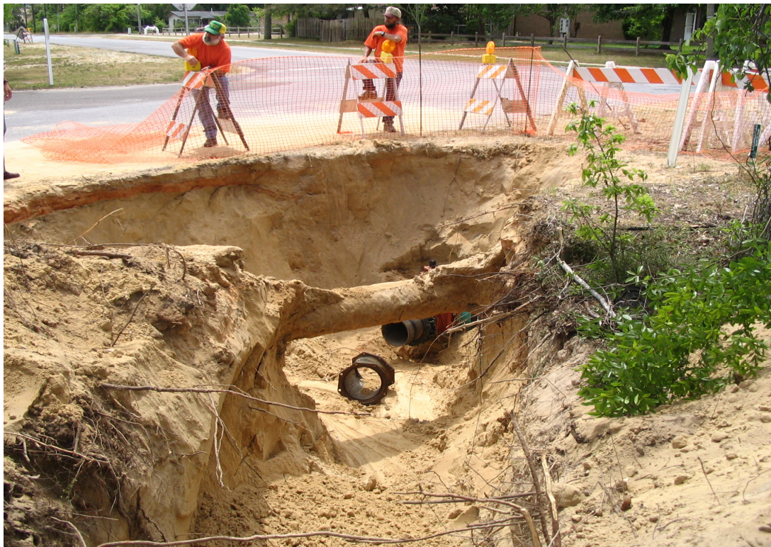
Old Line Removed, Ready for Installation of New Line
