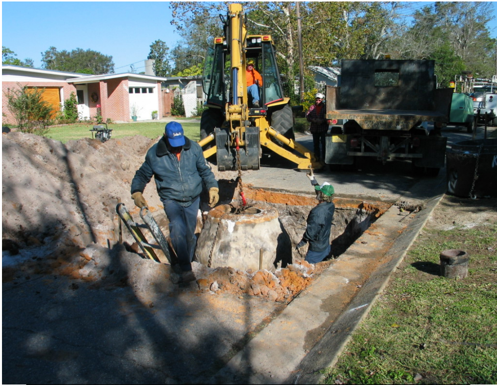
Replacing Sewer Line
