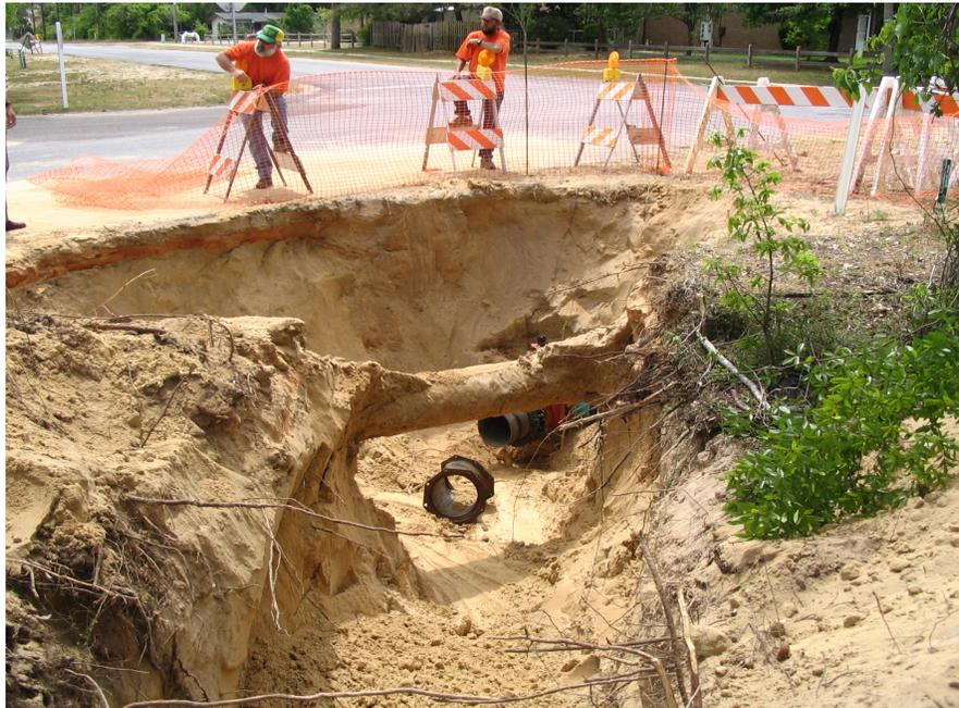
**Old line removed and ready for installation of new waterline**
