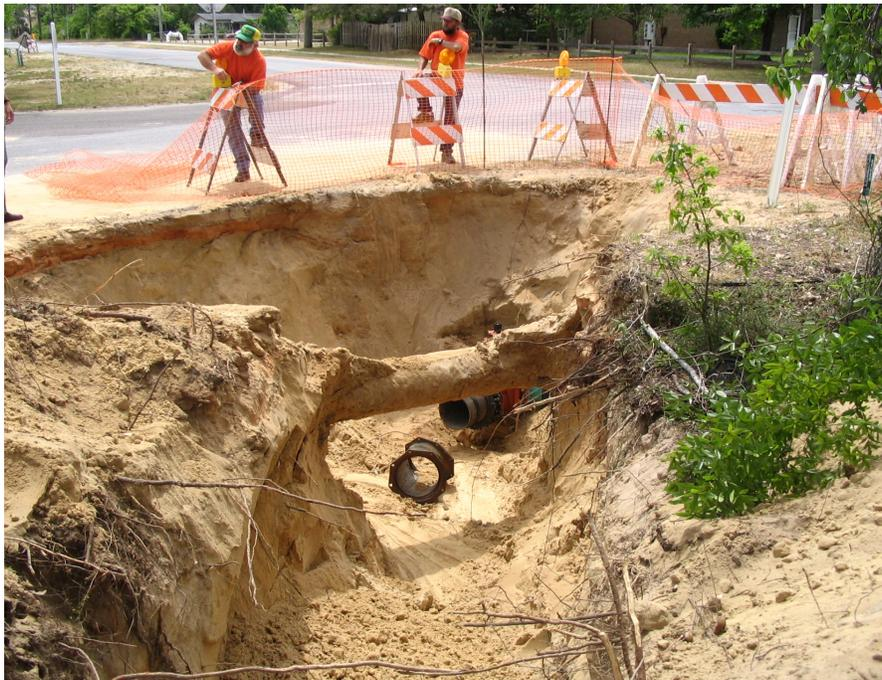
**Old line removed and ready for installation of new waterline**
